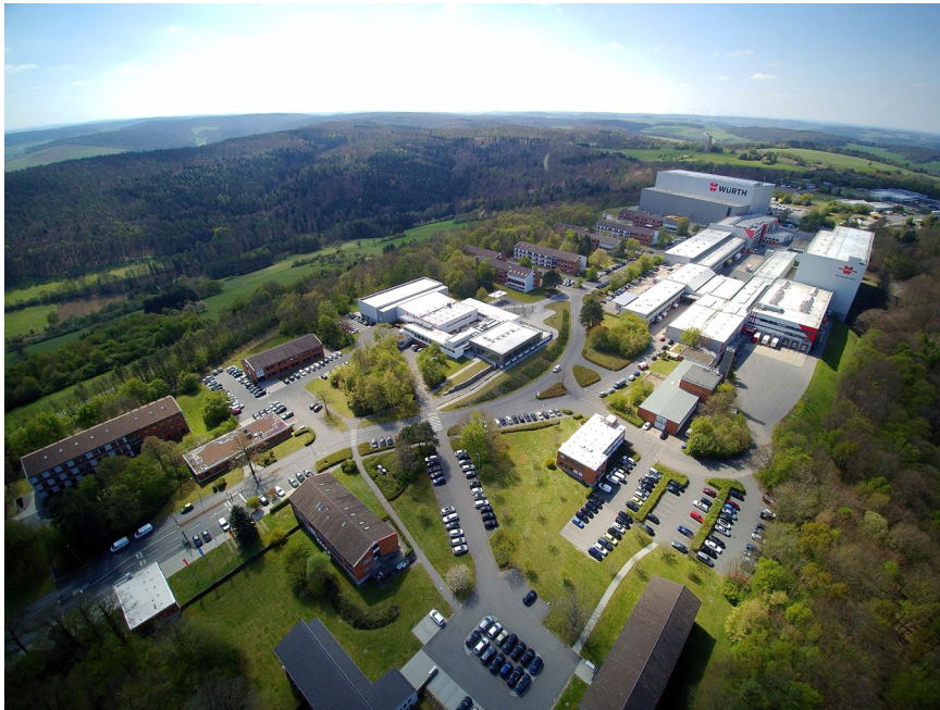
Photo 2: Aerial view of Würth Industrial Park.jpg
